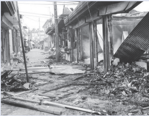
Private residence destroyed by North Korea's bombardment of Yeonpyeong Island |
